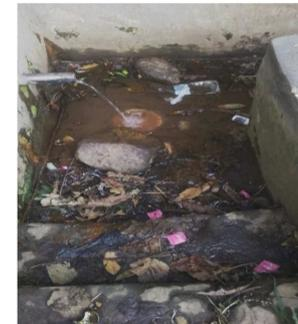
Figure 4. Protected spring water point showing potential sources of water contamination.
